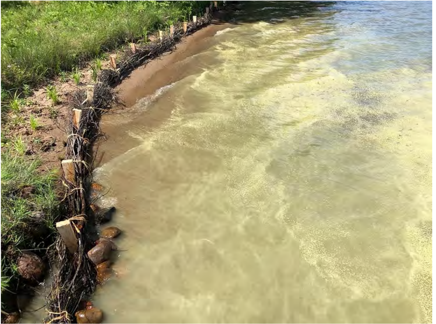
For places with more erosion, use multiple rows of willow as an additional barrier.
