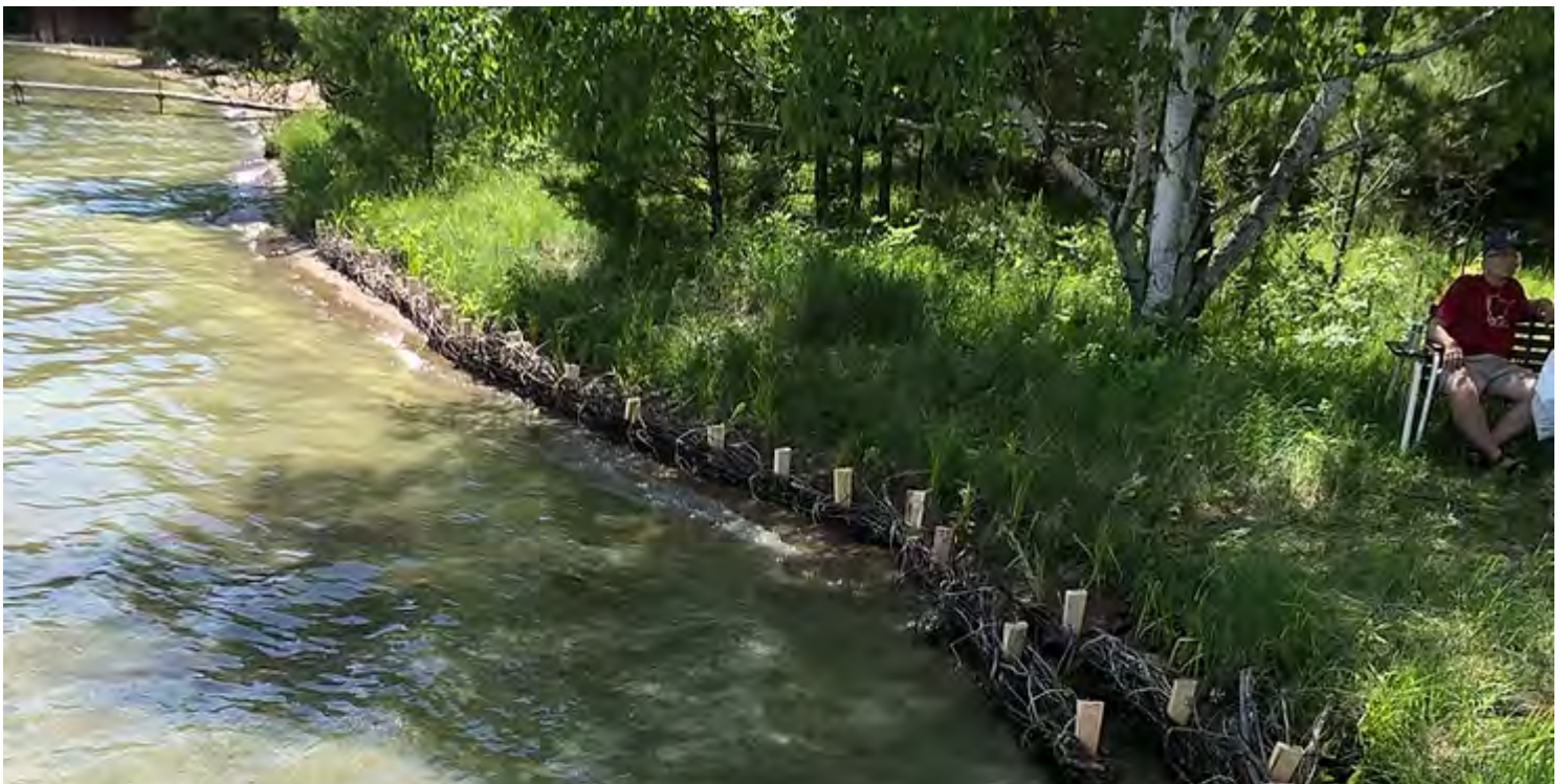
For places with more erosion, use multiple rows of willow as an additional barrier.
